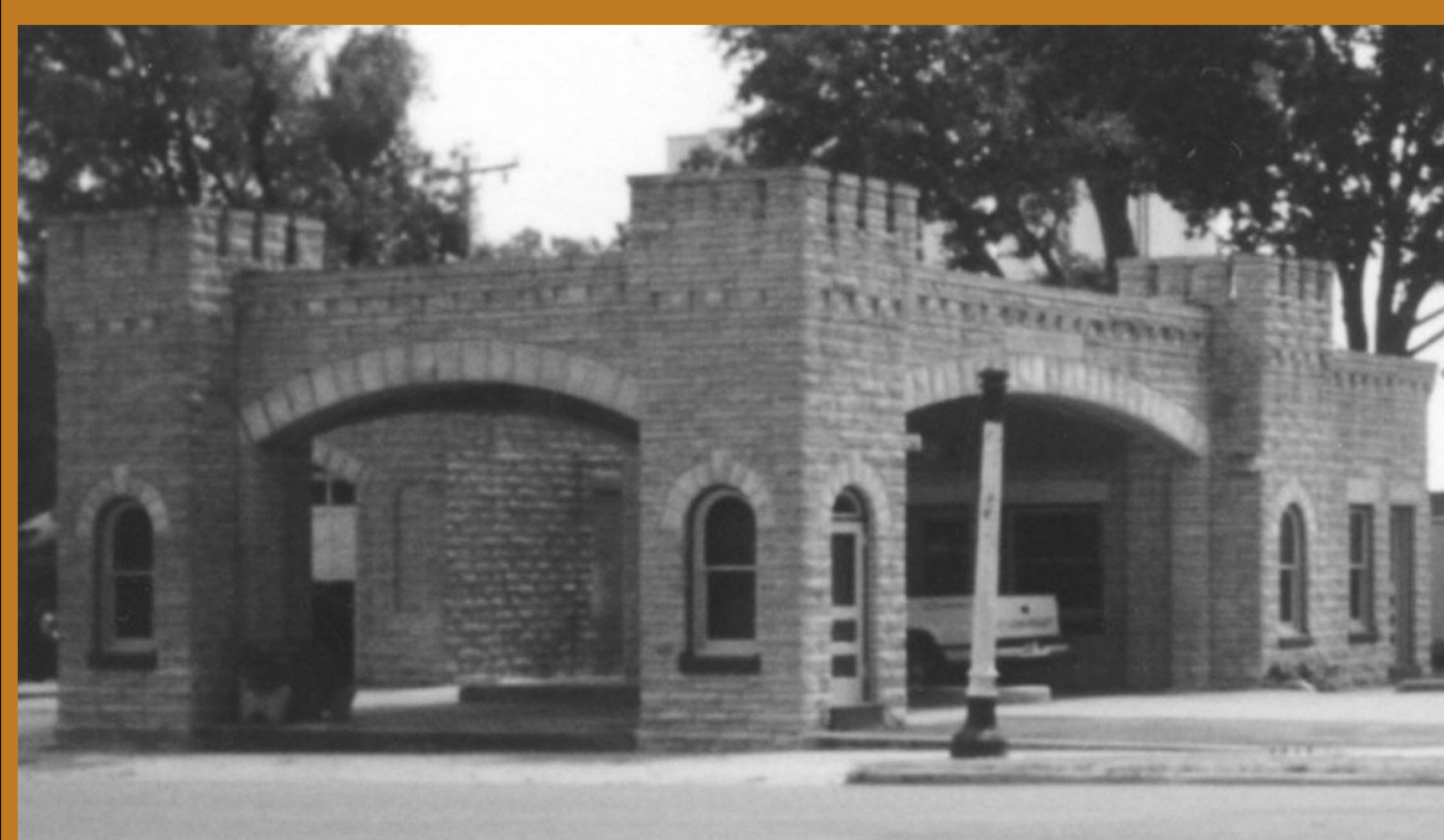
Glen Elder’s Castle Filling Station is listed on the National Register of Historic Places
