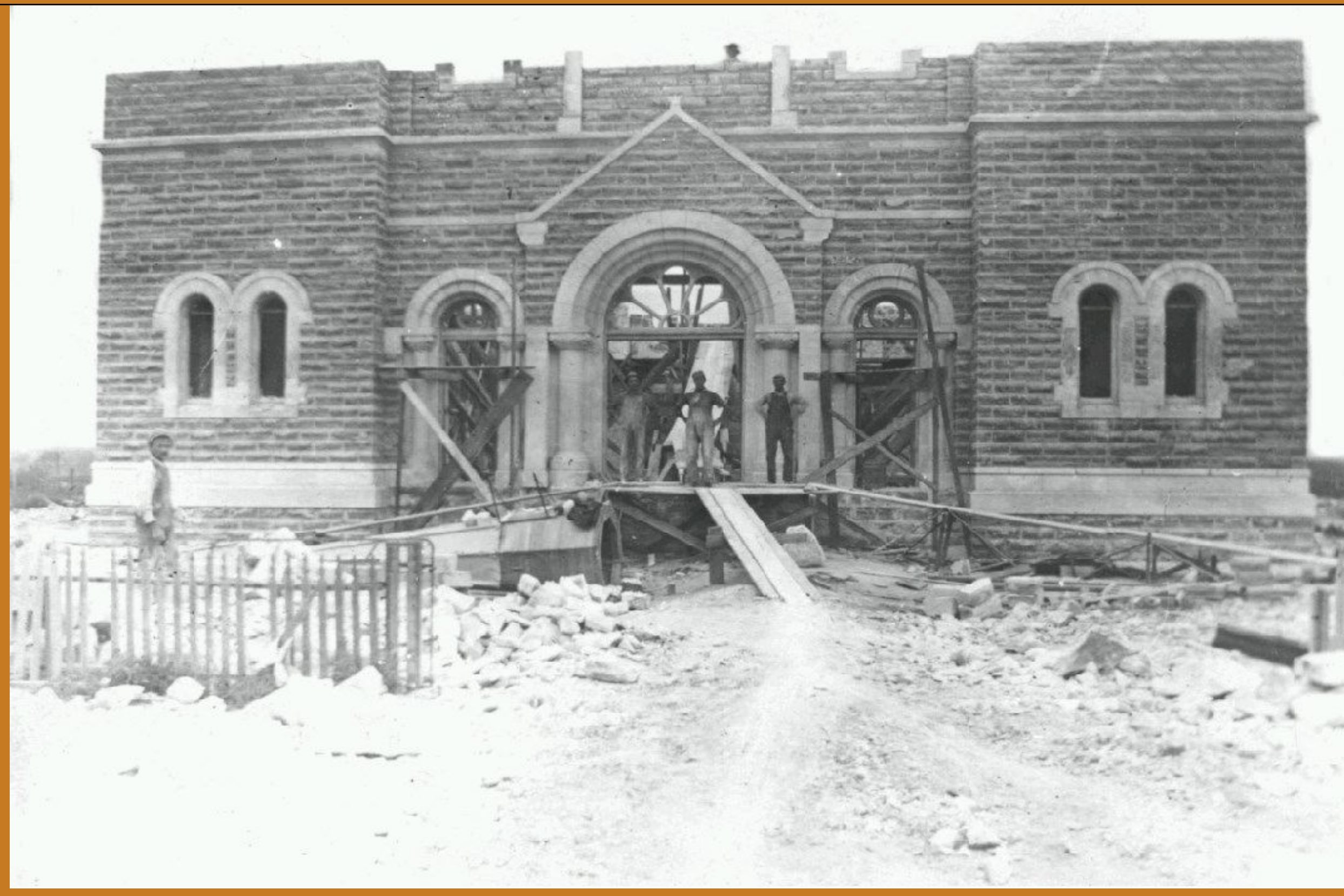
St. Joseph's Catholic Church under construction in Damar during the winter of 1911-1912.
